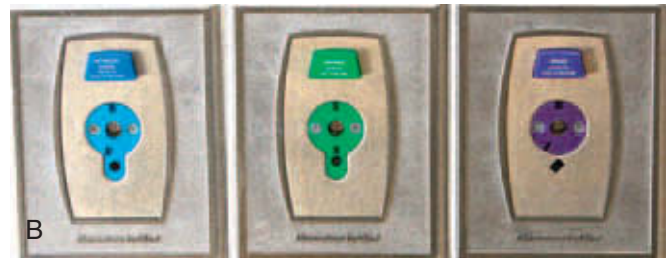
Figure 14-15 A and B, Diameter index safety system. Connectors attaching low-pressure tubing to inhalation sedation unit are of different diameters. O 2 (right) is of smaller diameter than nitrous oxide (left), thus preventing accidental crossing of attachments. (Courtesy James Soler.)
