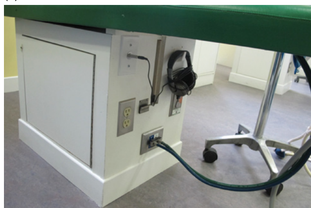
Figure 17-17. The custom bench can be made adjustable to seat a patient upright (a). It also can be designed with storage areas, and can contain video sound wiring and nitrous oxide/oxygen lines. Dimensions for the construction are contained in Box 17.1. Courtesy of Dr. Weinberger, London, ON, Canada.
